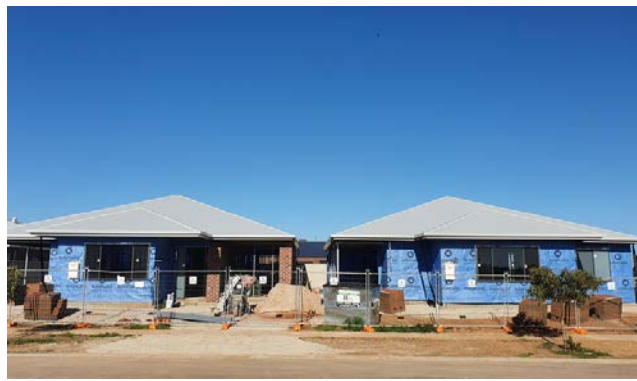
Houses wrapped and roof on
