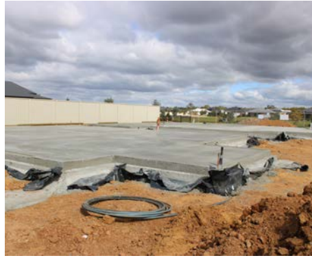
Poured slabs for both houses
