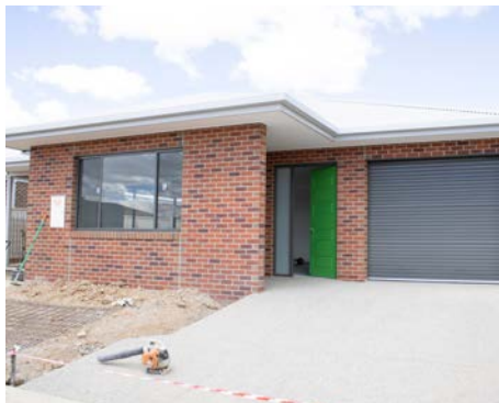
Driveways and doors painted
