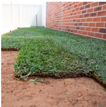
Grass being laid
