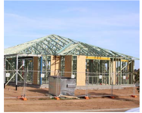
House and roof frame
