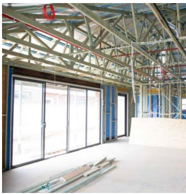
Electrical and internal work
